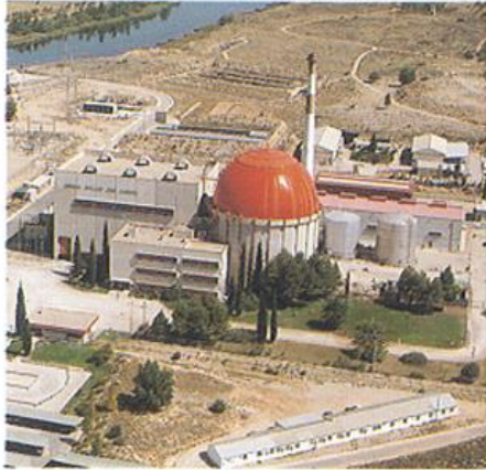
Jose Cabrera PWR – Westinghouse 160 MWe
