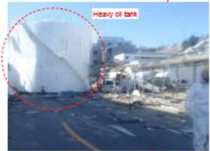
Heavy oil tank No major damage to the road, but the heavy oil tank carried by the tsunami blocked the road making it impassable. Photo taken 3/17
